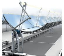
With the parabolic trough power plant, collectors concentrate solar energy onto a receiver tube positioned in the focal line and heat up the oil flowing in it. For high efficiency, all troughs have to be continuously adjusted to follow the sun's path and be focused exactly on the receiver tubes. This is achieved by magnetically coded position and angle measurement systems BML that are positioned directly on the rotating shaft.
