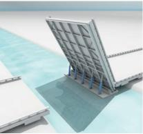
Every second counts when raising and lowering movable bridges, as impact on traffic must be kept to a minimum. High-precision position measurement systems integrated into the hydraulic cylinders ensure that the bridge raises and lowers quickly and efficiently. High-pressure resistant inductive sensors reliably identify the end position of the cylinder.
